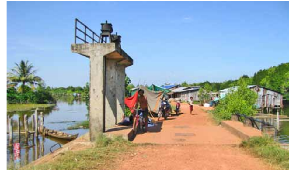
Prey Nub's water reservoir is 90 km in length constructed in 1930. In 1998, it was renovated and divided into smaller six blocks for better controlling. Nowadays, the second and sixth block need renovation as a result of a severe flood in 2009.
