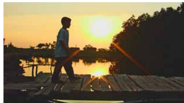
A kid is walking on the wooden bridge which is still under construction. This bridge also serves as a small port for them to tie up their boats.
